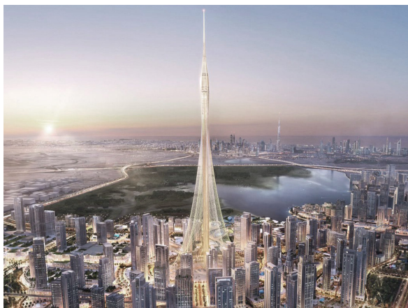
Dubai Creek Tower © Tom Evans
